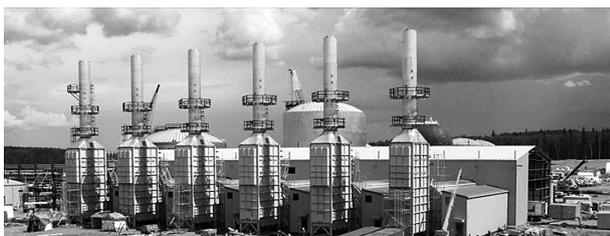
図12 SAGD Boiler (SAGD Facility) Skhneftegaz Engineering LLC
